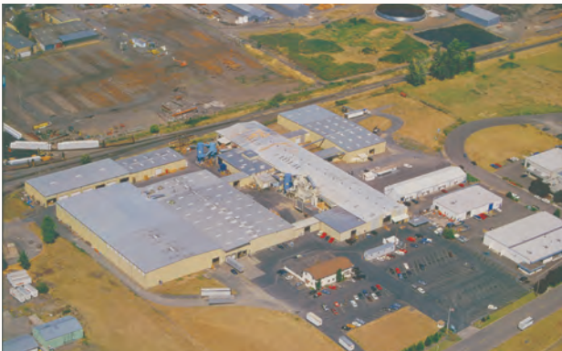
Whittier Wood Products Eugene manufacturing facility.
